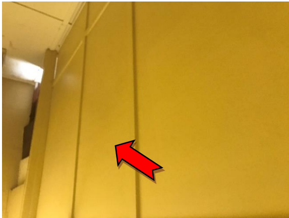
Photo 3. Interior, level 1, staircase, wall – asbestos-containing fibre cement sheeting.
