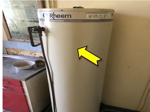
Photo 8. Interior, ground level, kitchen, hot water heater – suspected SMF internal insulation.
